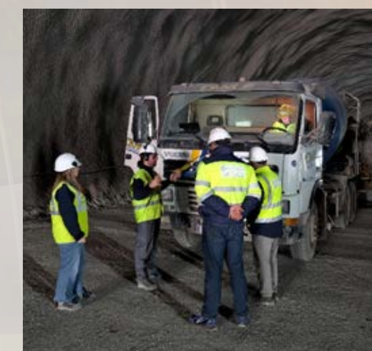
Tests carried out in the Tenerife Tunnel by FCC Construcción.
